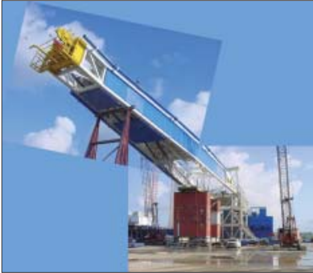
Parker Rig No. 262 mast rests on scaffolding in the construction yard at New Iberia, La. The rig's drawworks will upright the mast from the scaffolding, which will be the rig-up method at the Sakhalin drilling location (Fig. 11). Photo courtesy of ExxonMobil Corp.
