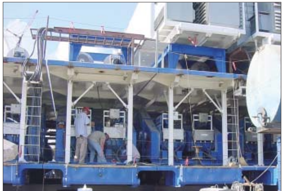
Power distribution equipment sits above the power generation sets, during construction in New Iberia, La. The drilling services module or utility train contains 50 skid equipment packages that must stack together for the module to fit within a reasonable space at the drilling location (Fig 10). Photo courtesy of ExxonMobil Corp.
