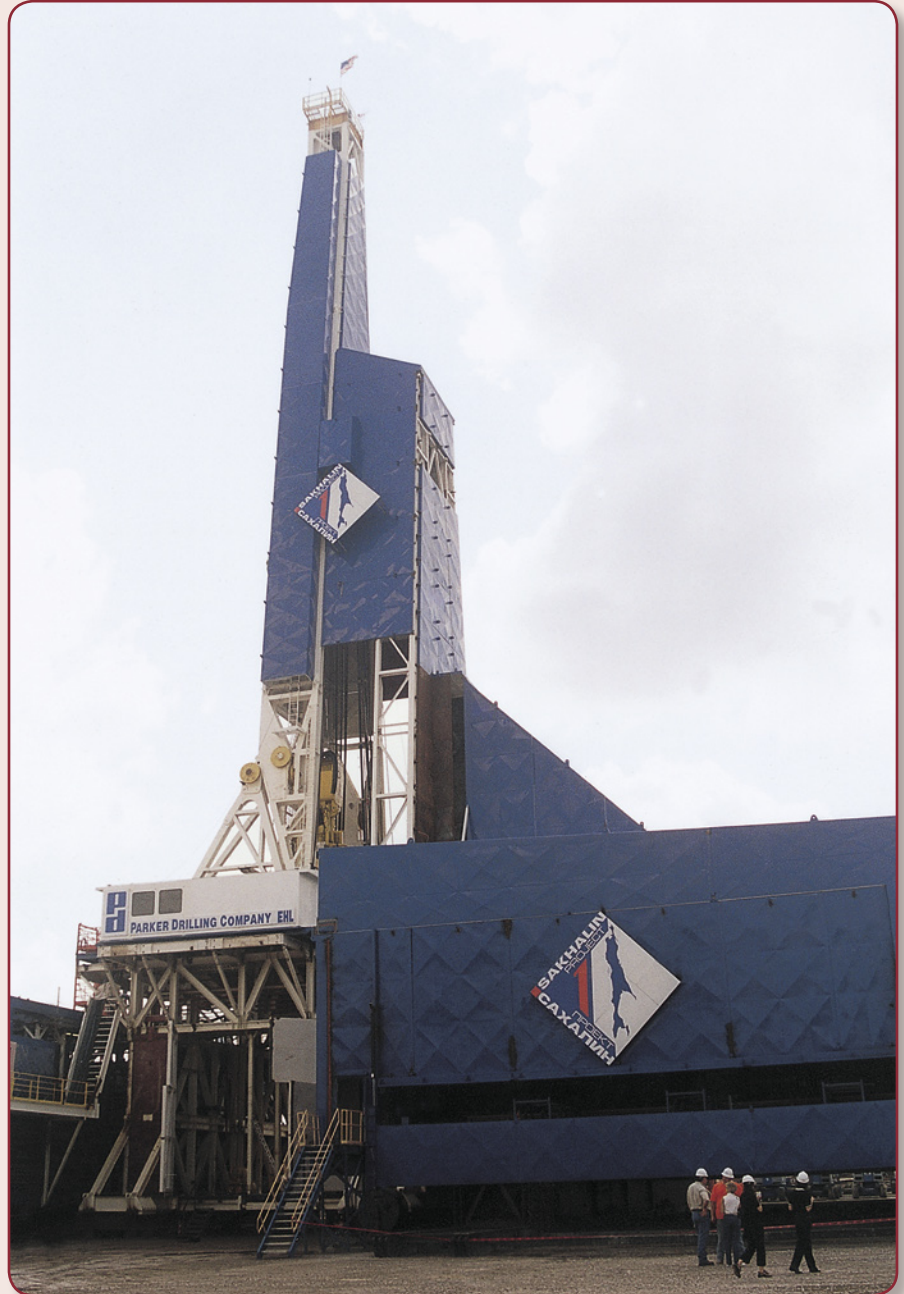
The Yastreb rig is shown in 2002 near the end of the construction phase in New Iberia, Louisiana. Parker Drilling designed, contracted construction and completed the rig in 18 months.
