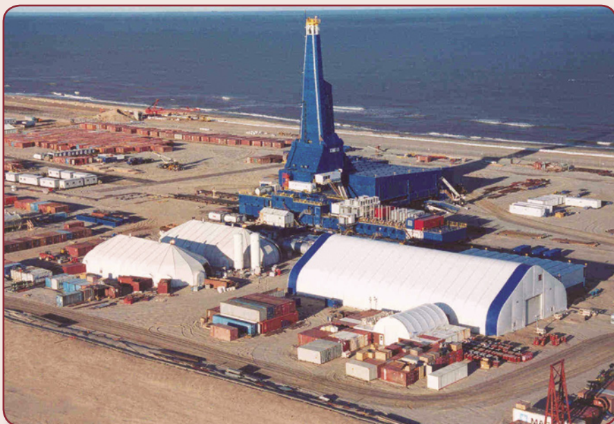
The Yastreb's first extended-reach well was initiated on August 8, 2004, and drilled to a vertical depth of three kilometers and a horizontal reach-out of 10 kilometers.
