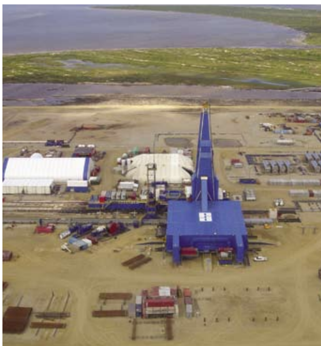
The Yastreb in Sakhalin Island, Russia. The rig is the world's largest and most powerful land rig and was constructed in New Iberia, Louisiana, for the Sakhalin-1 Consortium by Parker Drilling.
